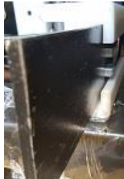
Figure: safety ladder installed into the cross beam. Note the safety latches extending past the ladder. The cross beam may need to be raised if the latches are to be moved for cable adjustment.
